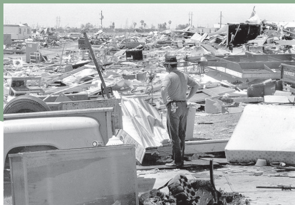
Surveying damage after Hurricane Celia. Source: Caller Times.
